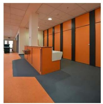
Skyline range is an extremely durable system and comes as standard with a 'P' section headrail, 'U' channel base rail and over-panel providing maximum stability.
